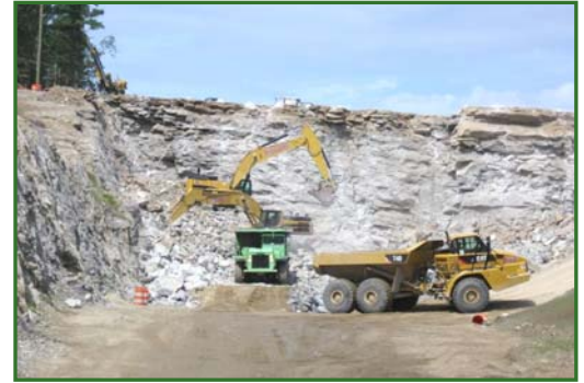
BLASTING & LEDGE/ROCK REMOVAL OPERATIONS
